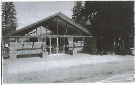
Malaghan Library extension, shortly after completion.
