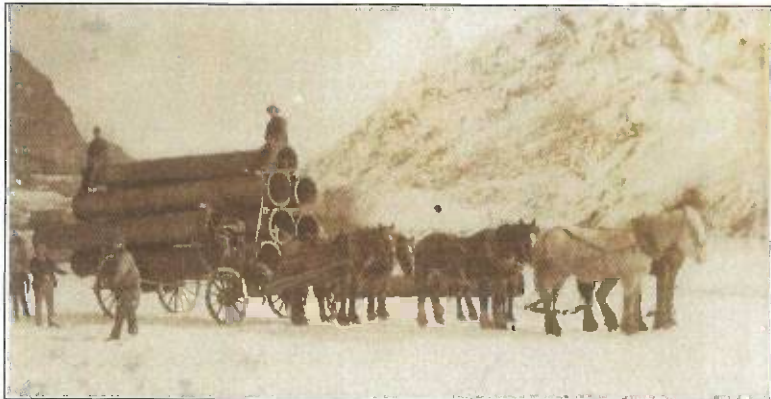
While the date of this photo on the Arrow Flats is uncertain, it is likely the pipes are destined for Bush Creek.
